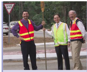
With the Mayor Cr Reade Smith, and Cr Jarman at the intersection of Stanley's Road and Red Hill Road which is being upgraded thanks to Commonwealth Roads to Recovery Funding and the Mornington Peninsula Shire Council.
