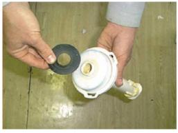
If water is not overflowing into the overflow tube, the leak is associated with the outlet valve. You will either need to replace a faulty washer or install a new cistern outlet kit. Firstly, turn off the supply tap that delivers water to the cistern and flush the toilet so the cistern is empty. Unscrew the complete outlet valve from
