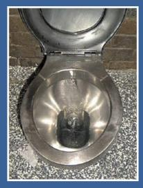
To work out how much water or money is actually being wasted; press an empty cream container (200ml) against the back of the bowl where the leak is coming down. After one minute see how full the container is and estimate the volume gathered. The chart below provides an estimate of annual water wastage and its cost.
