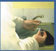
Finally, screw the aerator back on to the tap head.
