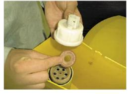
Firstly, turn off the supply tap which delivers water to the cistern and flush the toilet so the cistern is empty. Unscrew the inlet valve so the faulty washer is revealed. Take the washer to the hardware store to ensure that the correct size replacement washer is chosen. Replace the inlet valve with the new washer and re-assemble. Turn the supply tap back on, wait for it to refill and ensure the leak stopped.
