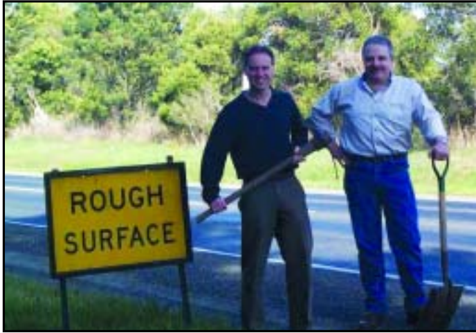
Greg Hunt with local resident Neale Burgess working to deliver on the now completed upgrade of the Western Port Highway slipway.
