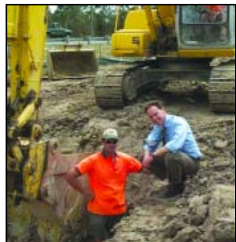
Greg with construction workers upgrading the Western Port Highway
