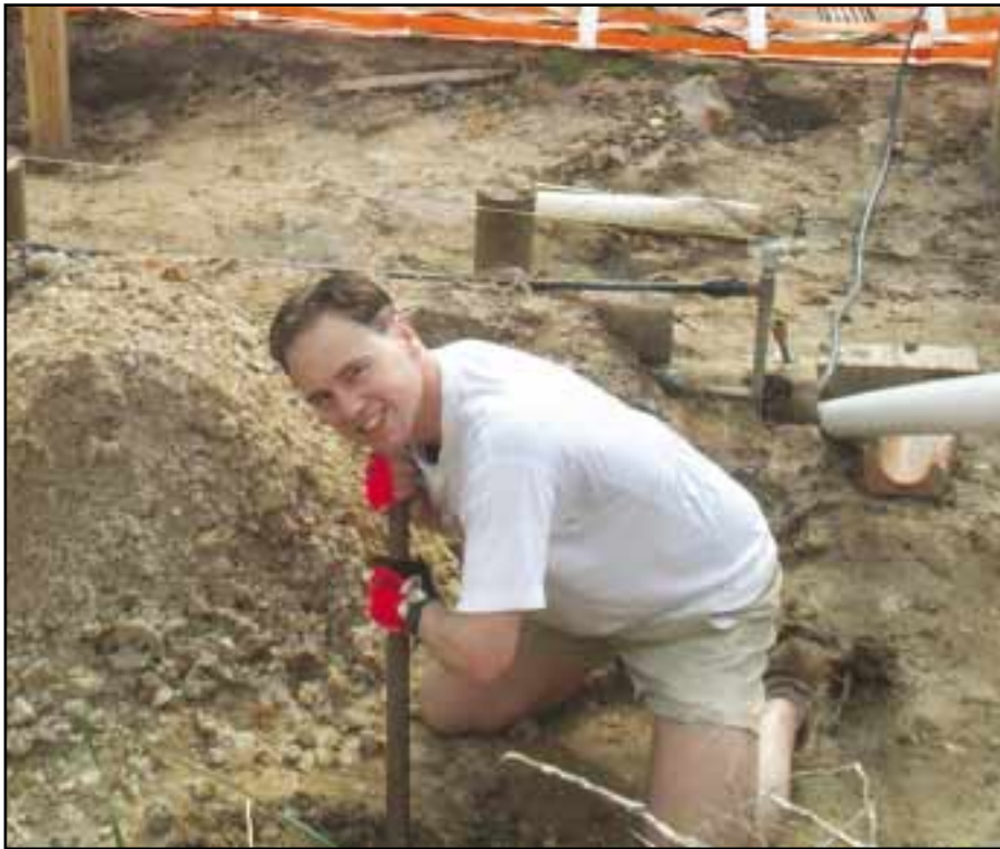
Greg helping dig foundations at the Mt Martha Bowls club
