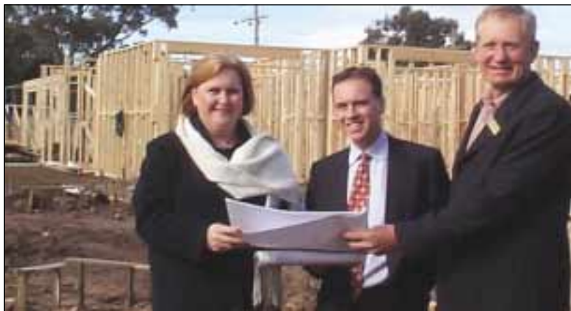
Greg Hunt MP examines construction of the new wing of the Regis Grange Aged Care Centre in Rosebud with Manager, Judy Kelly and Development Manager Denis Mathieson.
